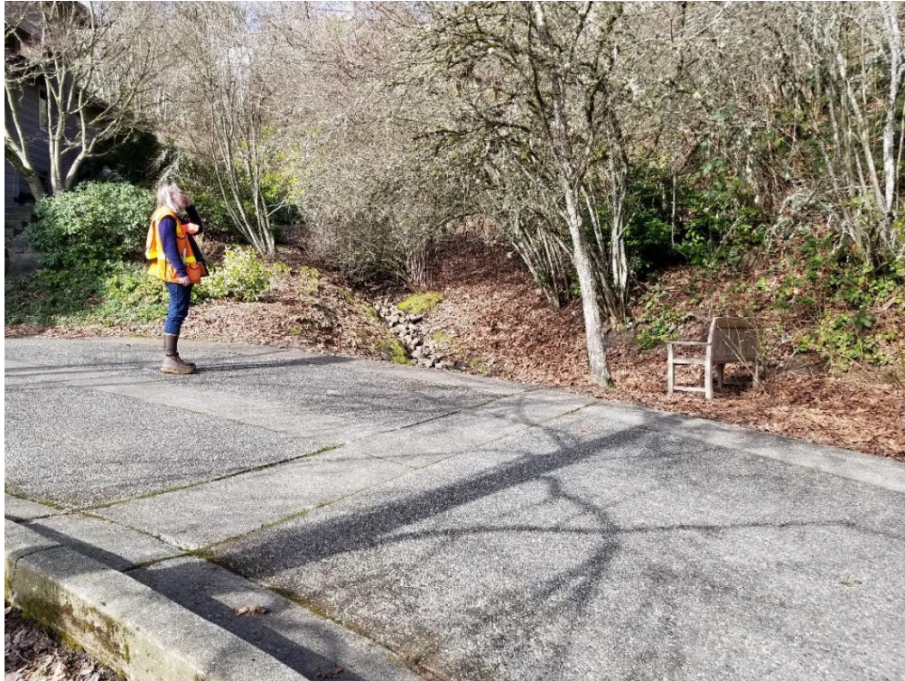
Photo 11—Driveway to 7511 92 nd Avenue Southeast. The stream channel is conveyed under this driveway by a culvert.
